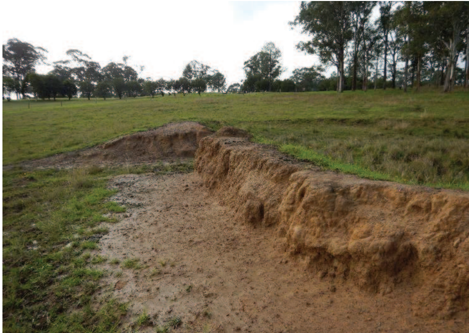
Figure 9: Eroded dam wall in Survey Unit 2 showing soil exposure. View north east.
